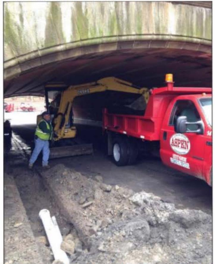
Aspen crews, saw cutting the roadway, installing 8" main water pipe and then installing irrigation followed by landscaping in Central Park NYC.
